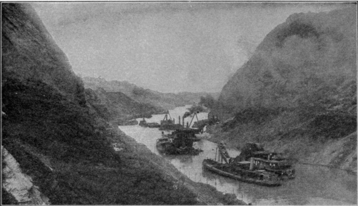
CUCARACHA SLIDE ATTACKED BY A FLEET OF DREDGES
