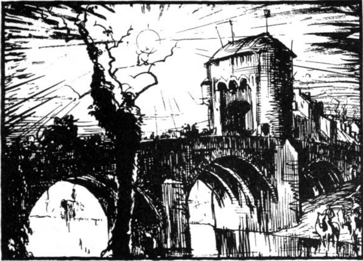
WAR-BRIDGE AT MONMOUTH
