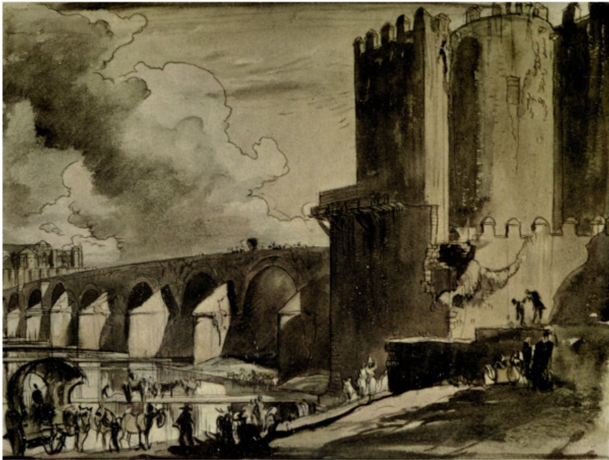
THE HUGE DEFENSIVE BRIDGE AT CÓRDOVA IN SPAIN. ORIGINALLY ROMAN, BUT REMODELLED BY THE MOORS IN THE NINTH CENTURY, RECENTLY SO MUCH REPAIRED THAT LOOKS ALMOST NEW
