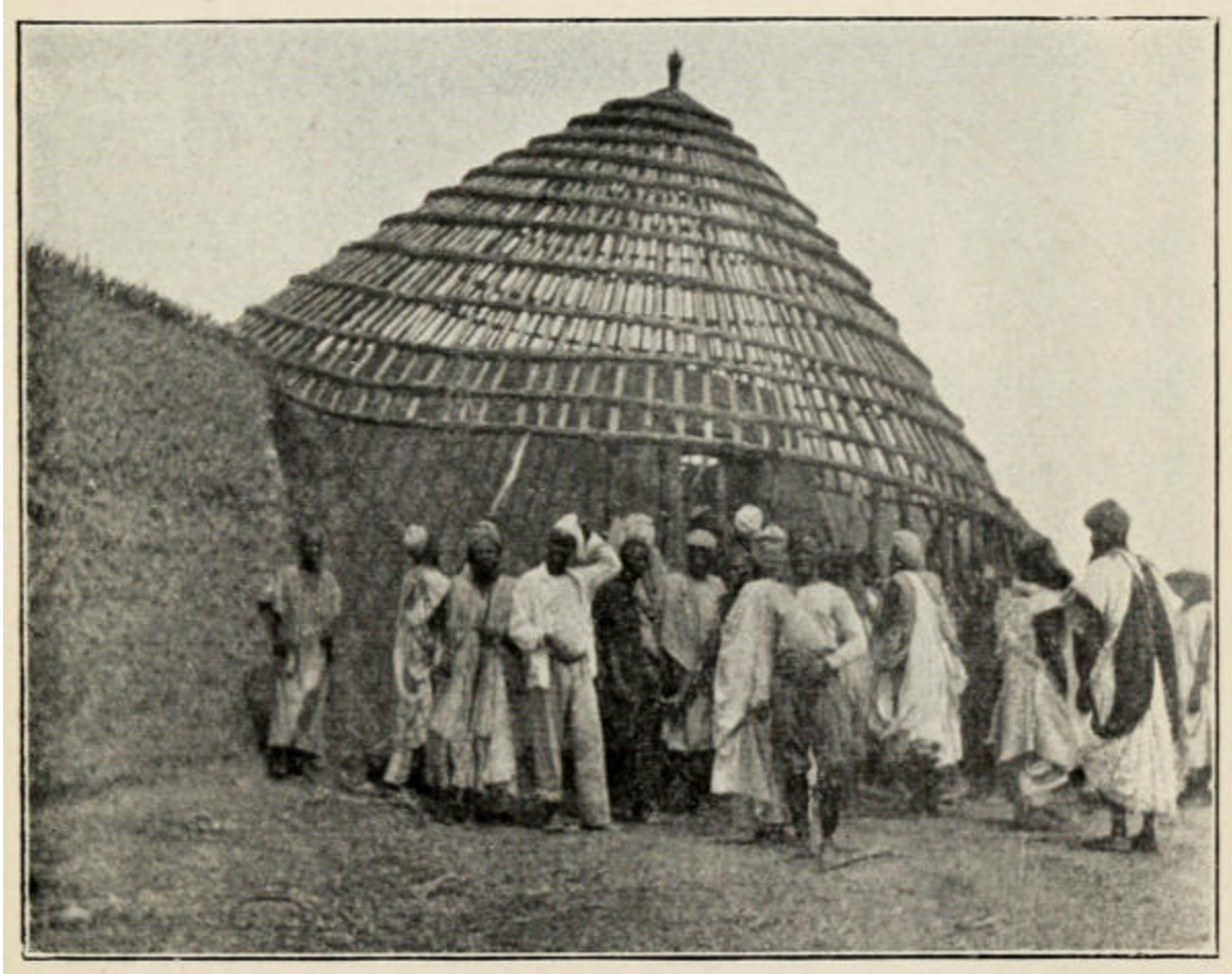
ROOFING AT KEFFI. (p. 51)
